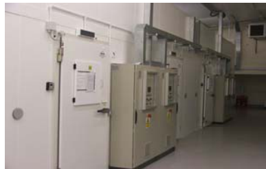
Containment rooms B63
