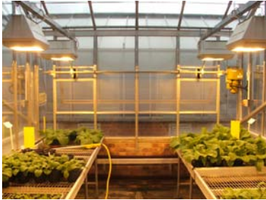
Compartment in G34, naturally ventilated, showing Phillips 400 watt SON-T lamps
