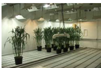
Cereal Growth Room. (R19) Note automatic watering & HQI lamps in the room.
