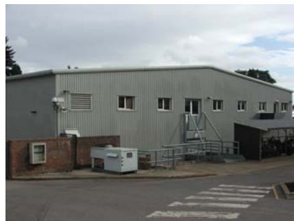
CE building (B57)
